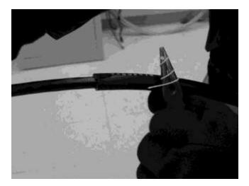
Figure 10 – Pull the ripcord through the armor and outer jacket.
