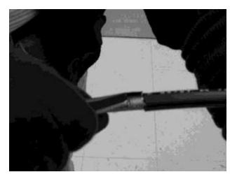
Figure 6 - Lift and separate the armor at overlap.
