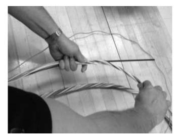
Figure 52 – Cut the central strength member in multiple steps while unwinding the buffer tubes.
