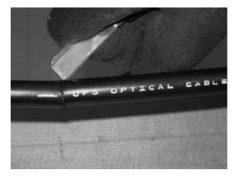
Figure 24 - Make a longitudinal cut between the two closely spaced ring marks.
