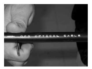
Figure 22 – Ring cut the cable jacket.
